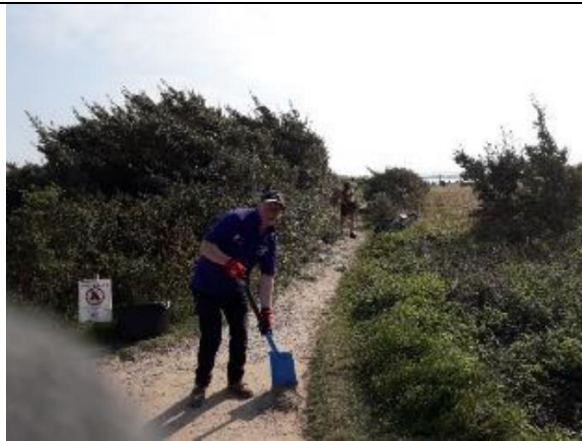
Path work at Chanonry Point with volunteers to improve disabled access
