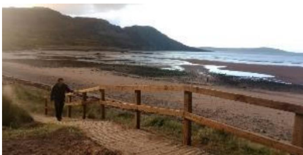
Installed a handrail at Gruinard to prevent dune erosion
