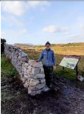
Rebuilt a dyke at Durness, prevents off-road parking
