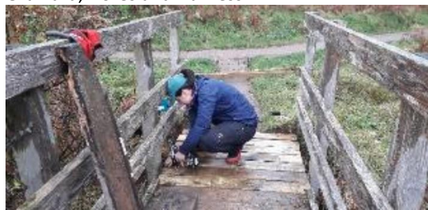
Repairing a bridge at Gairloch
