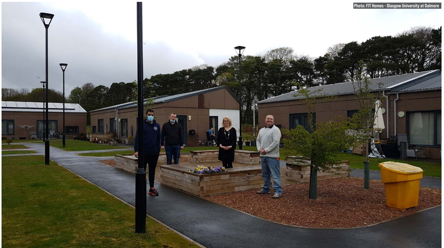
Photo: FIT Homes - Glasgow University at Dalmore
