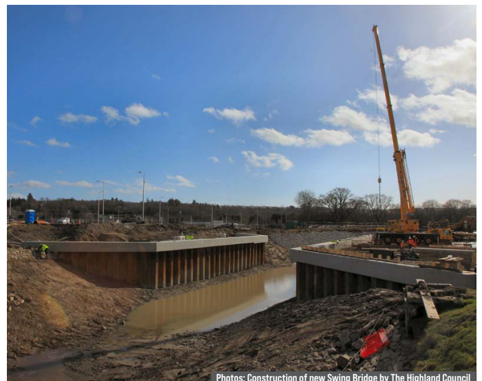
Photos: Construction of new Swing Bridge by The Highland Council
