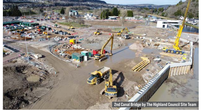
2nd Canal Bridge by The Highland Council Site Team
