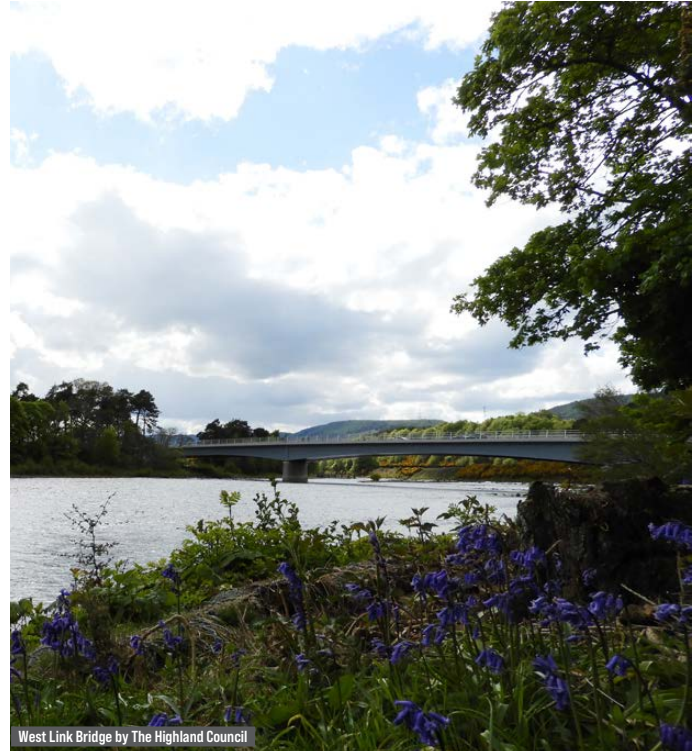
West Link Bridge by The Highland Council
