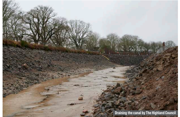
Draining the canal by The Highland Council
