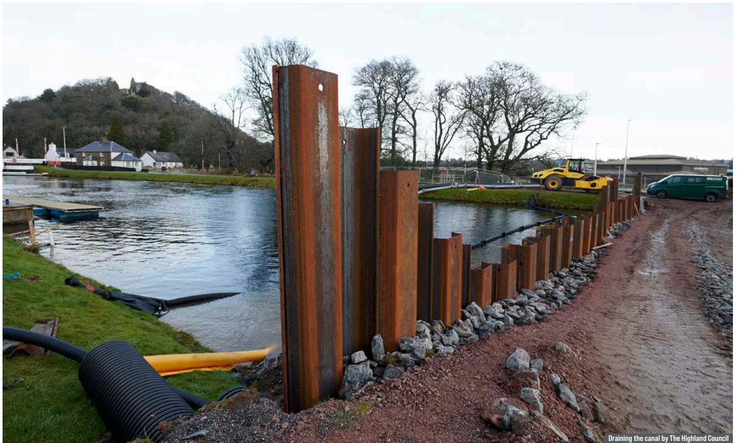
Draining the canal by The Highland Council
