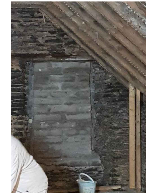
Image - Existing blocked up first floor window from inside.
