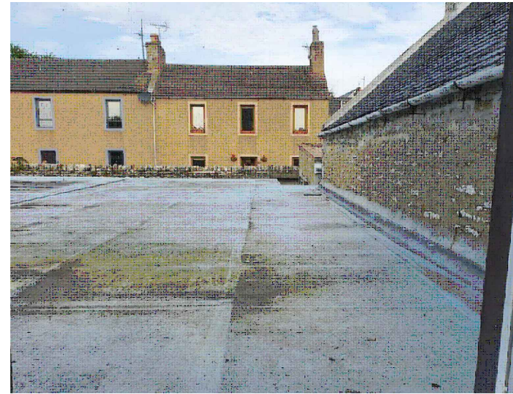
IMAGE - Existing flat roof and stone wall.
