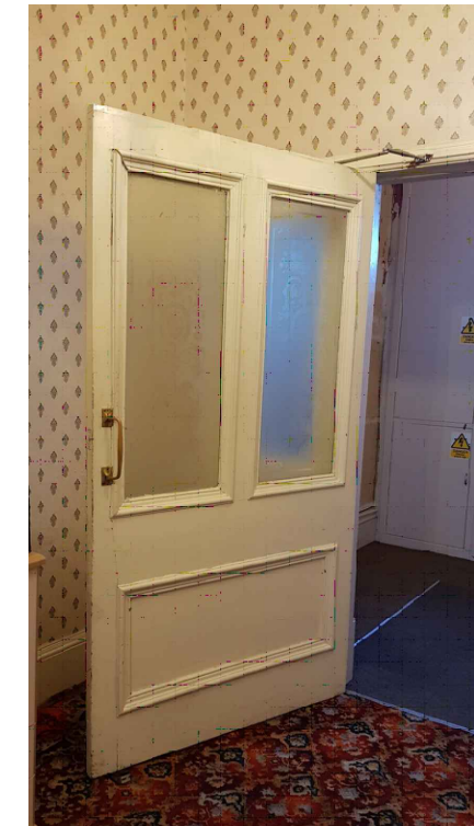
IMAGE - EXISTING GR. FLOOR LOBBY DOOR
