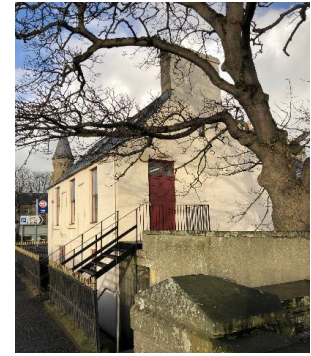
Thurso Bridge/Riverside Road Buildings
