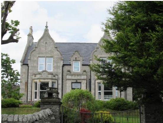
Springbank House, Janet Street
