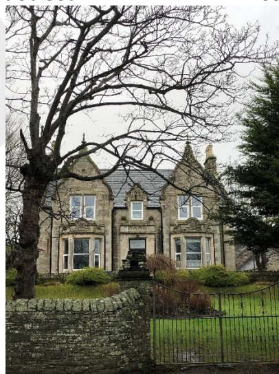
Springbank House, Janet Street
