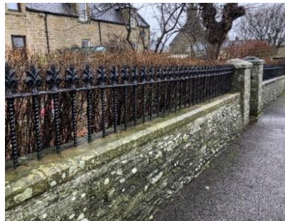
Detail of traditional cast iron railings
