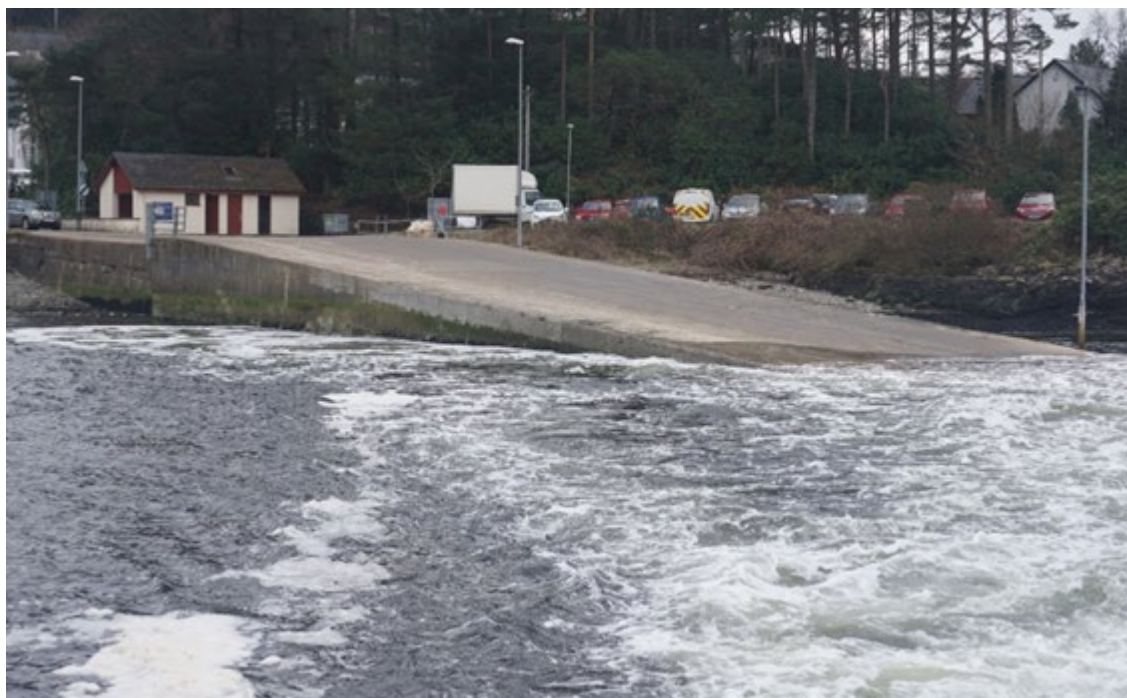
Figure 2.3: Nether Lochaber Slipway
