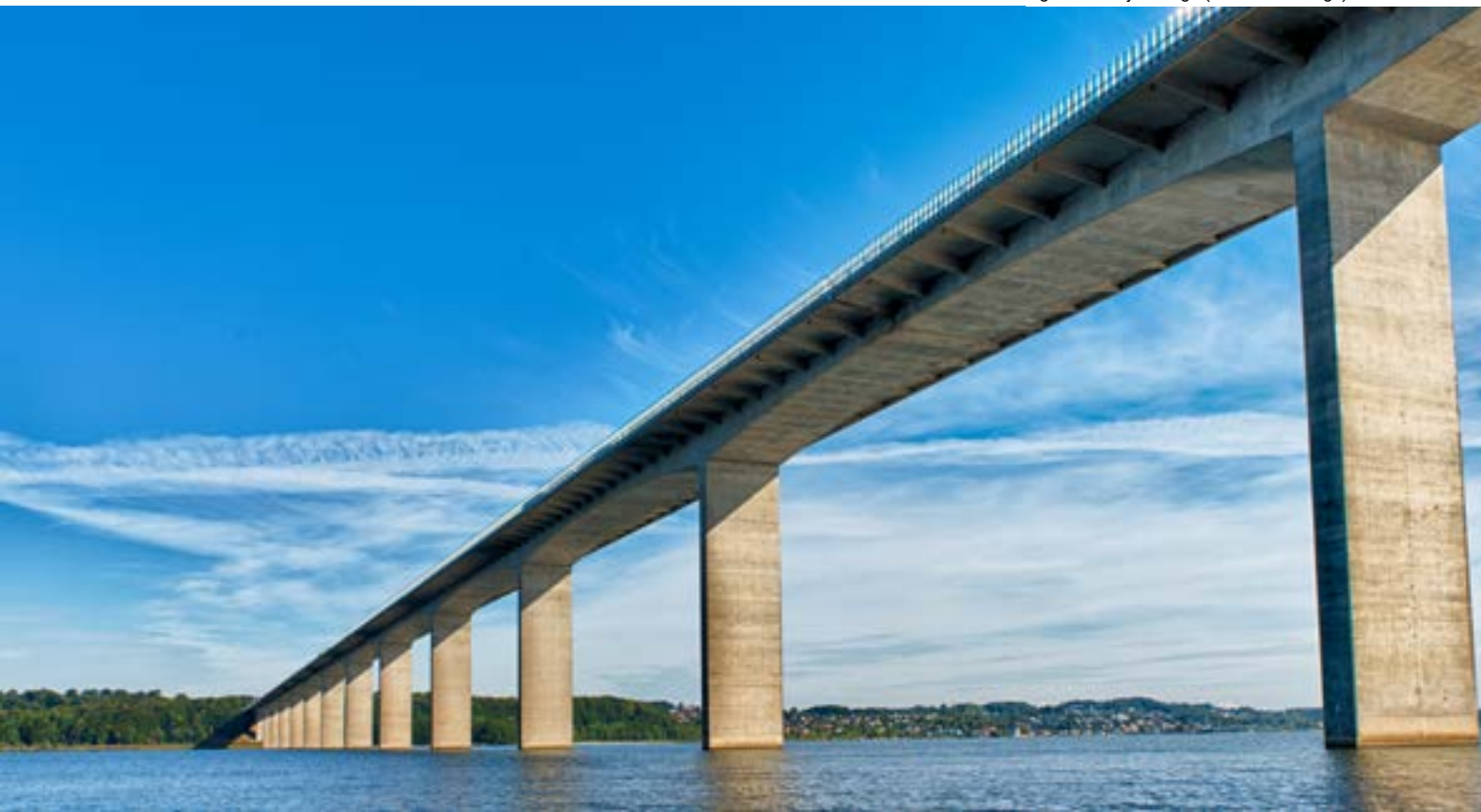
Figure 21: Vejle Bridge (Cantilever Bridge)
