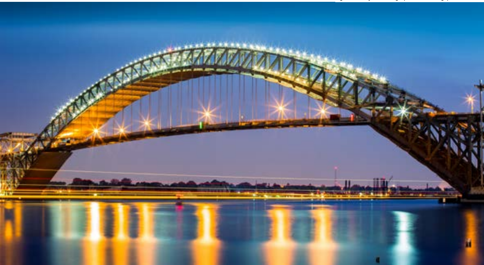
Figure 19: Bayonne Bridge (Tied Arch Bridge)
