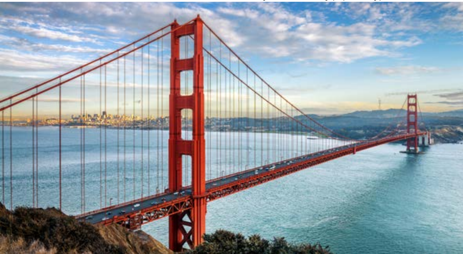
Figure 18: Golden Gate Bridge (Suspension Bridge)
