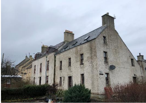
Miller's Lane, category B & C Listed buildings
