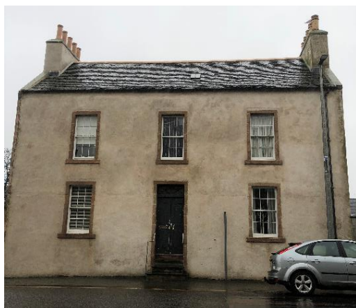
Traditional lime mortar harling
