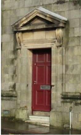
Doorway with pediment
