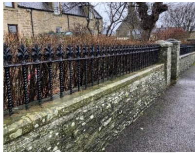
Detail of traditional cast iron railings
