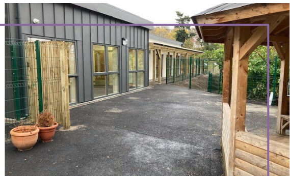
• Avoch Primary, Exterior Nursery Unit
