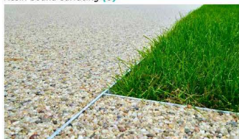
Resin bound surfacing (3)
