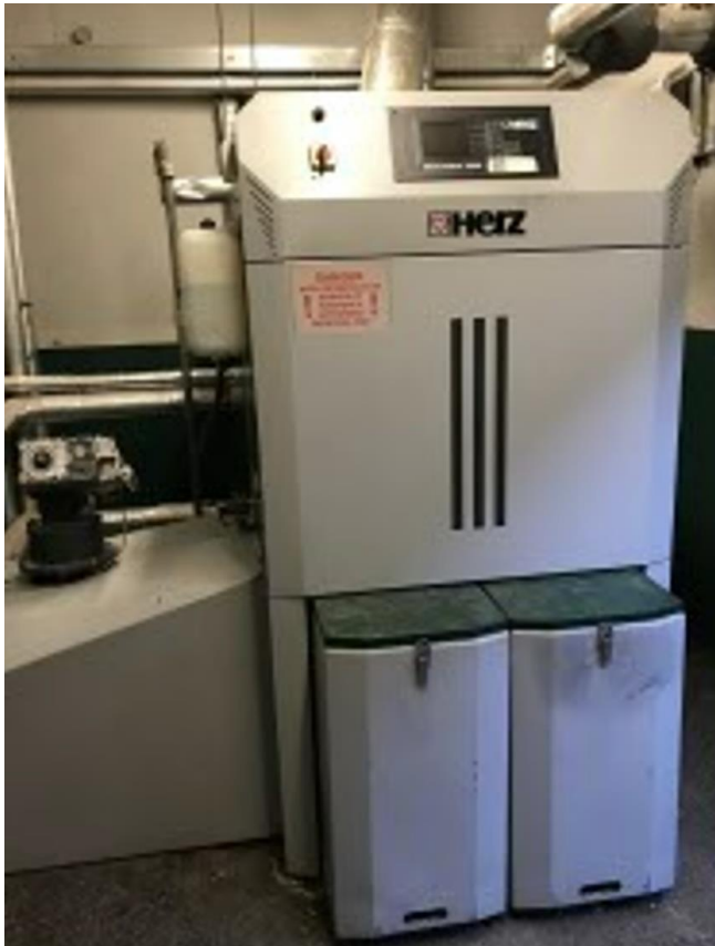
Figure 4-15 Biomass boiler in container unit, adjacent to west wall
