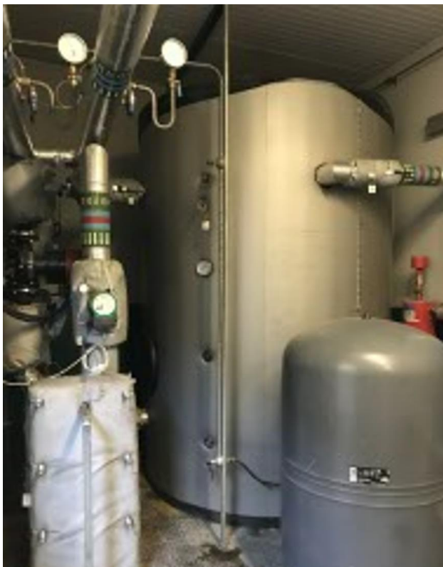
Figure 4-15 Biomass boiler in container unit, adjacent to west wall
