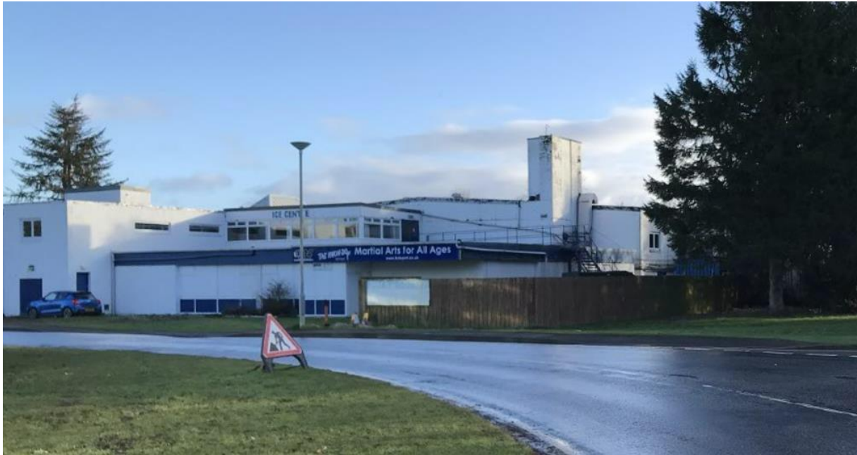
Figure 4-27 Inverness Ice Centre, view looking north-east
