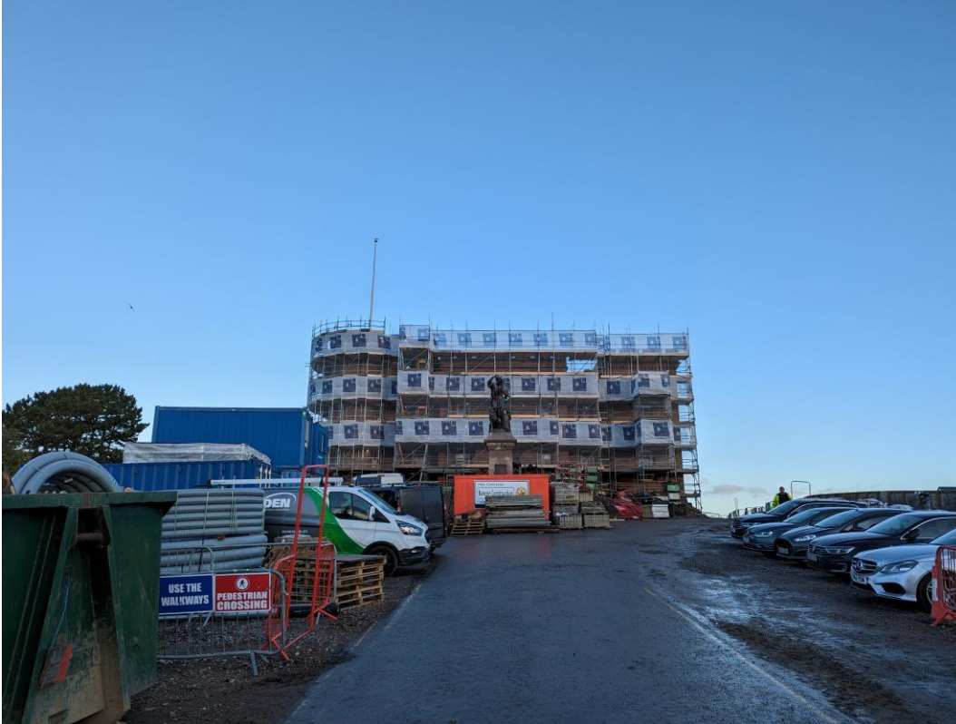
Figure 4.1: Inverness Castle during refurbishment works
