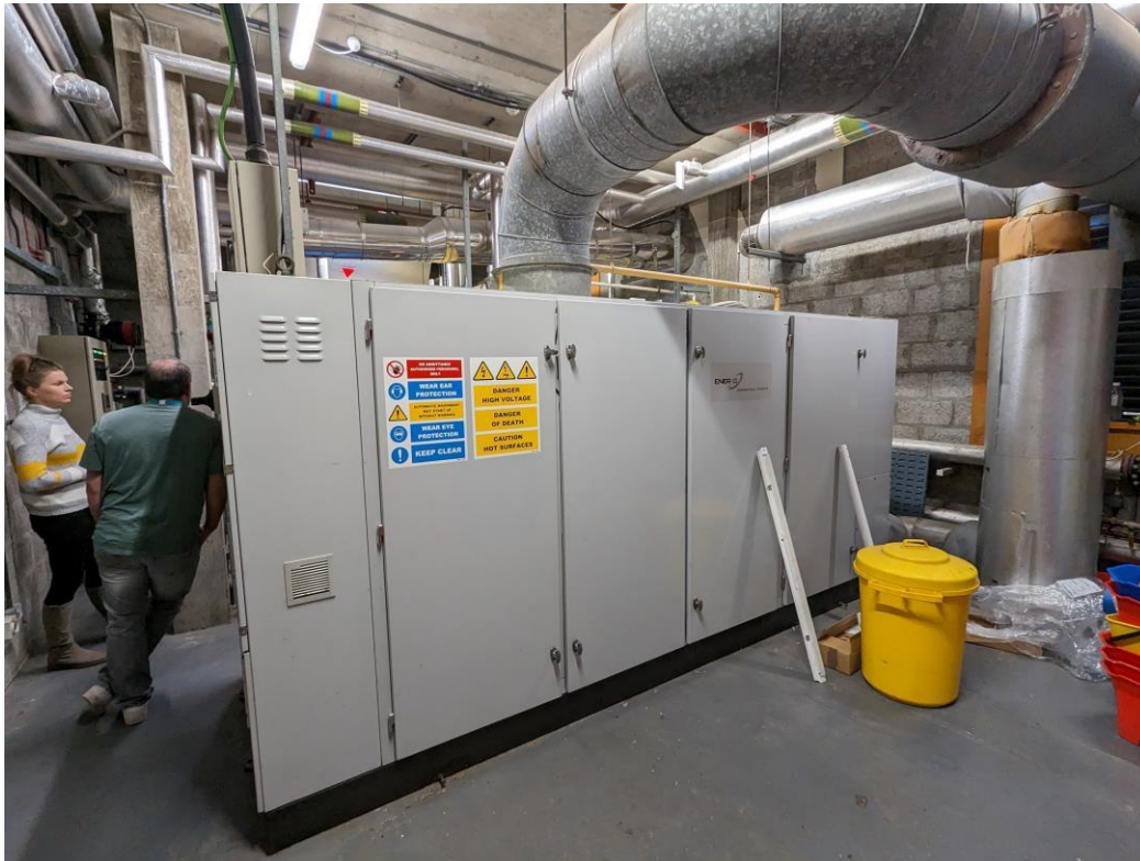
Figure 4-3: Wet side CHP unit - retired
