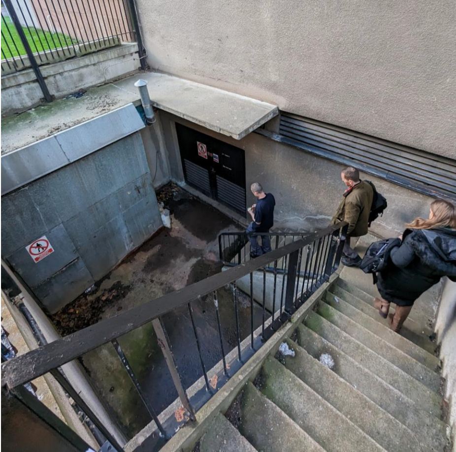
Figure 4-6: Basement level entrance to the Highland HQ energy centre
