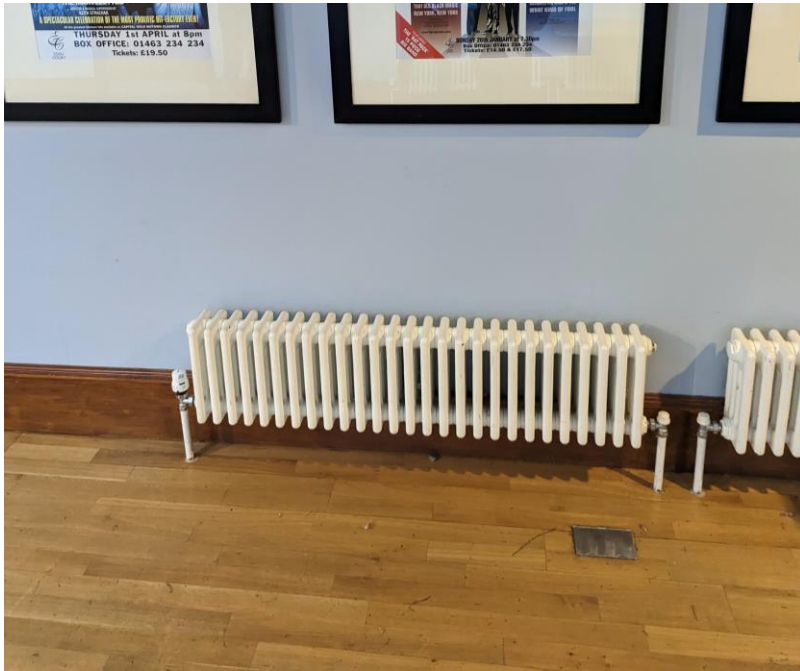
Figure 4-30: Wet radiator space heating
