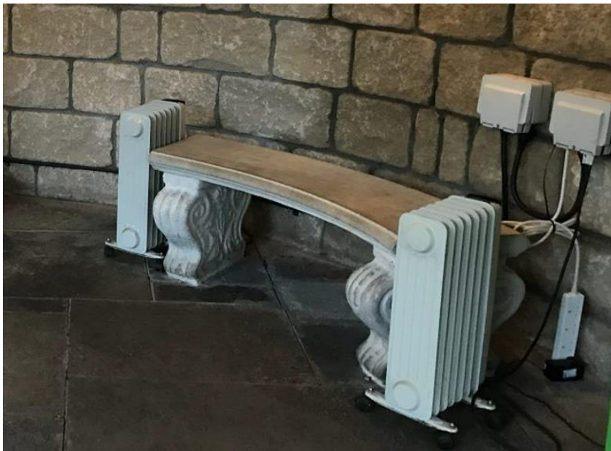
Figure 4-22 Glass greenhouses, backup electric heaters (oil-filled)
