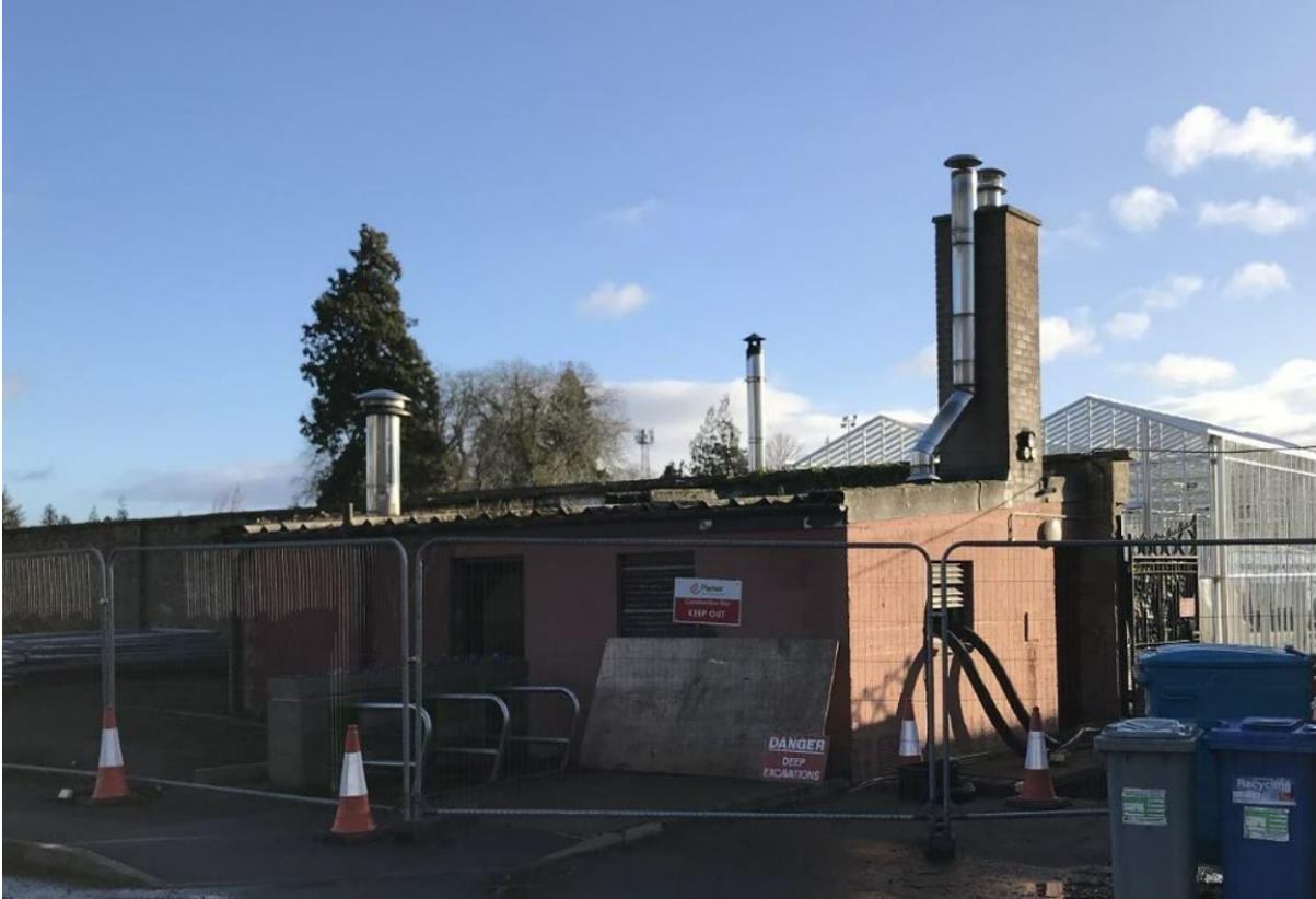
Figure 4-11 External plantroom housing gas boilers, West side of site
