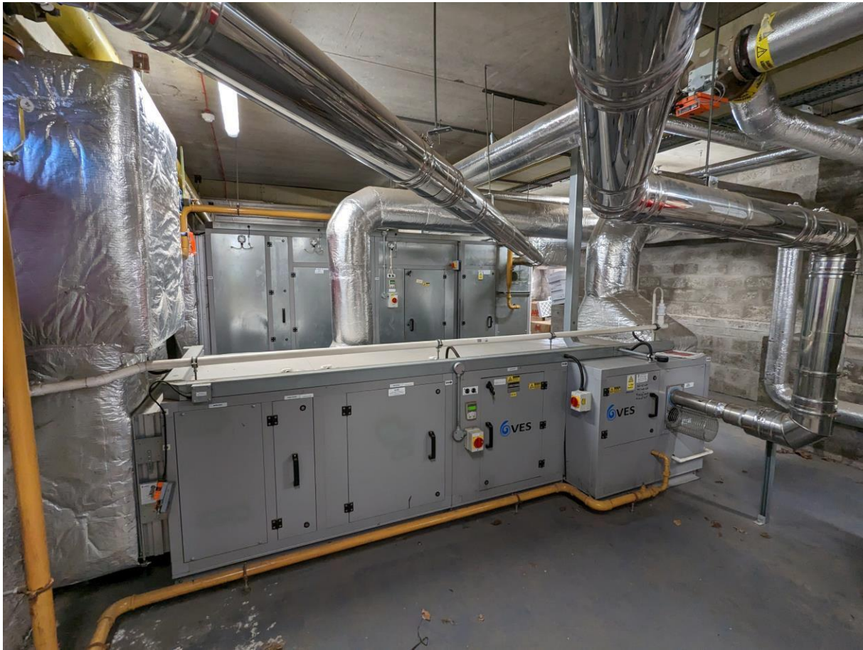
Figure 4-2: Dry side gas fired heaters - small unit in foreground and large unit in background
