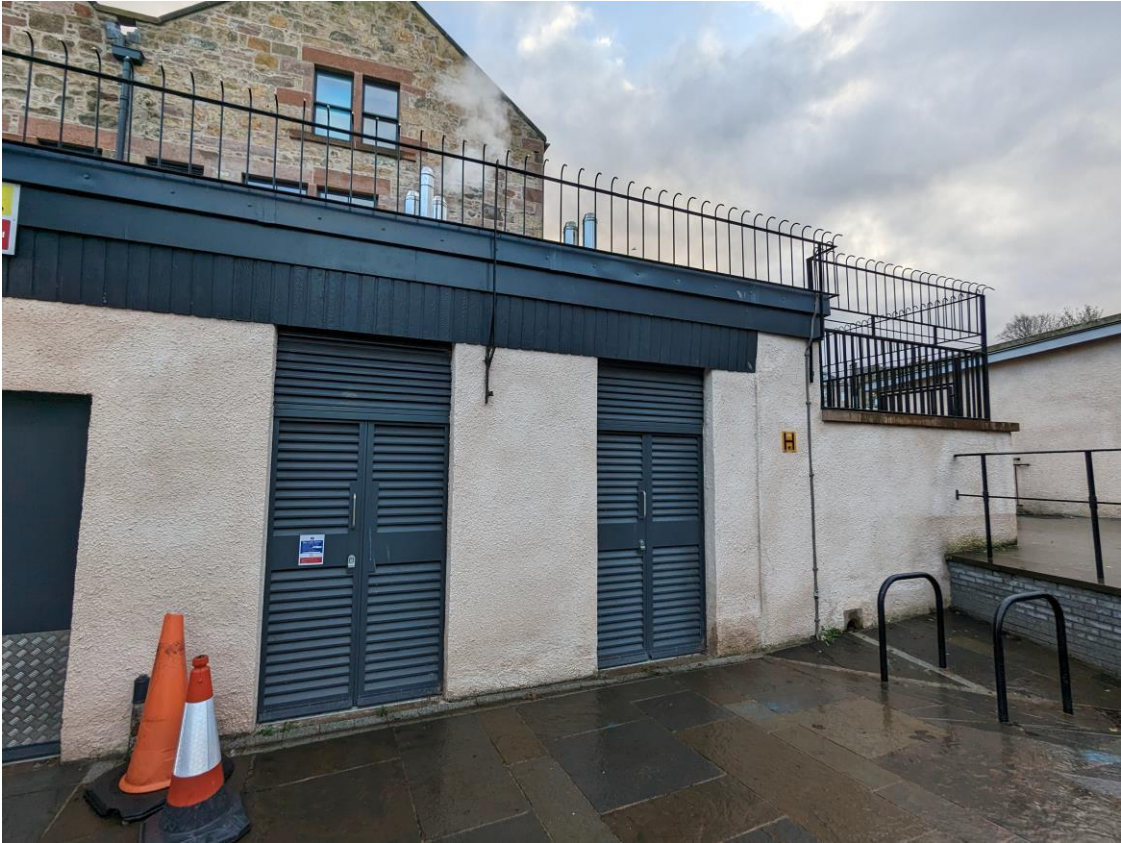
Figure 4.7: External facing doors to the boiler room
