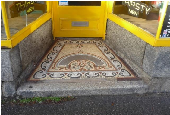
Traditional shopfront design often incorporated a lobby, and its threshold may display decorative tiles or trade names which are increasingly rare and should always be retained.
