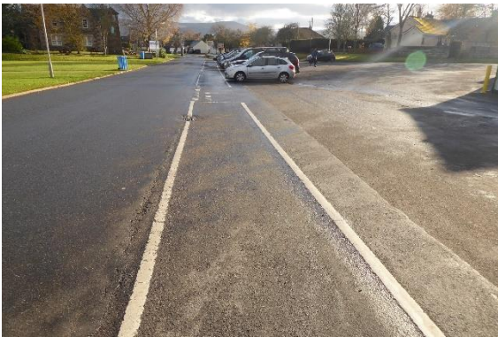
Pedestrian route from Castle Road through Burnfield Avenue is only defined by lines on the tarmac.
