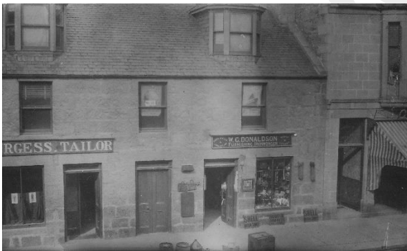
In a number of buildings, earlier ground floor opening patterns have been altered for example by combining /relocating / widening doors and windows which chiefly effects the symmetry and fenestration pattern of the traditional parent buildings and groups of similar buildings.
