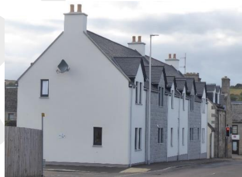
Recent flatted development using architectural elements such as pitched dormers, chimneys, copes and contrasting wall materials to articulate the street façade and provide a characterful design. The building height has been matched well to the neighbouring traditional building.
