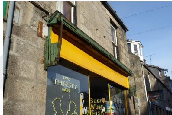
Traditional retractable blinds were popular in Grantown and several shops retain blind boxes and mechanisms.
