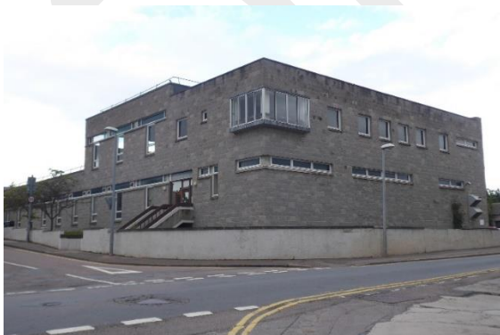
General view from the Telecoms building.
