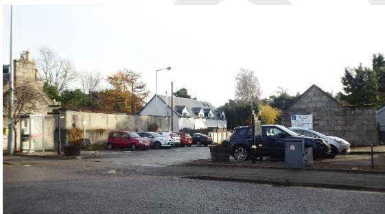
Loss of boundary definition at the south High Street carpark where buildings previously lined the street.
