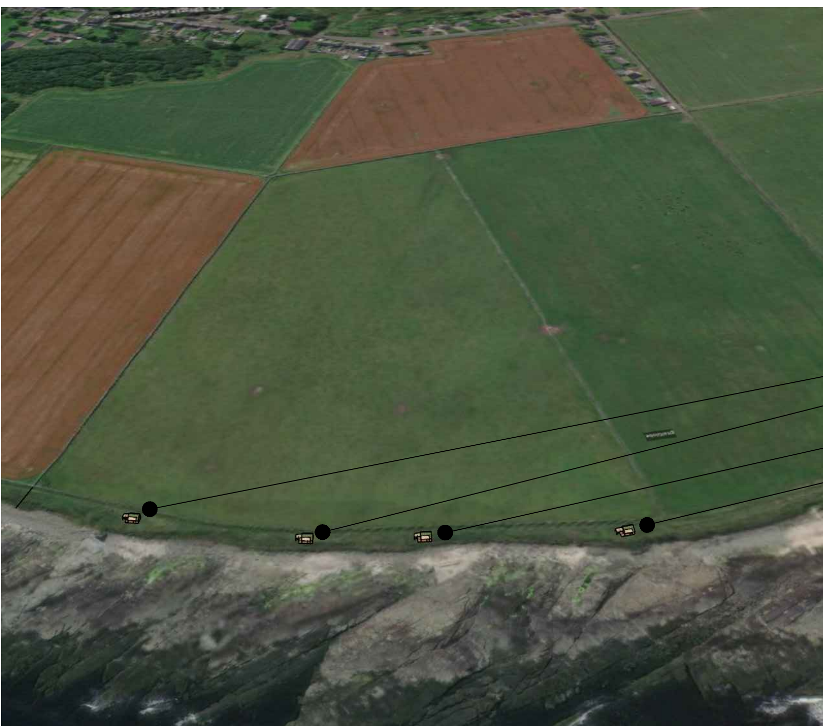
04 G10 AERIEL VIEW FROM NORTH
