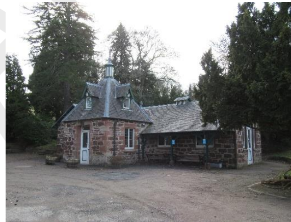
Fig. 27 Upper Pump Room
