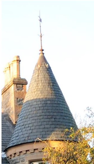
Fig. 50 Turret and finial detailing
