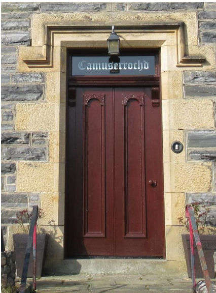
Fig. 45 Single leaf, double panel door with sign-written top light
