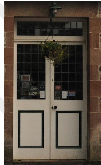
Fig. 47 Double leaf, half-glazed and moulded panel door with multi-pane top light
