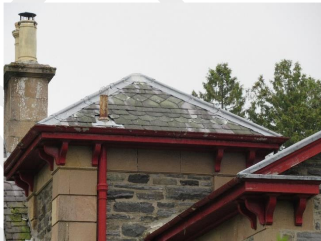
Fig. 38 Fish-scale and diamond slate tiling detail
