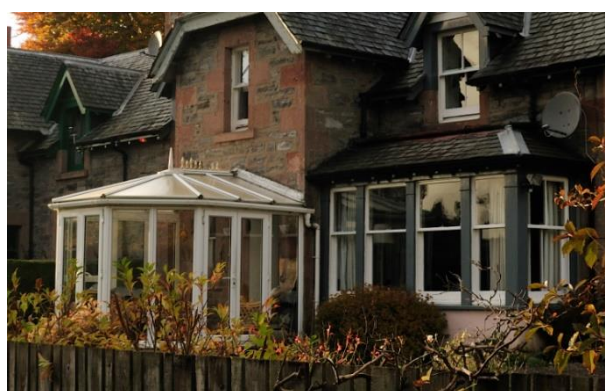
Fig. 70 Inappropriate conservatory extension
