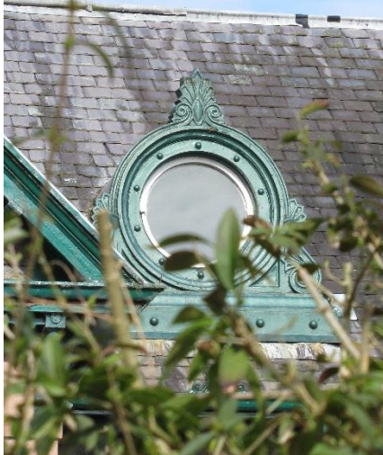
Fig. 42 Ornate cast iron dormer window
