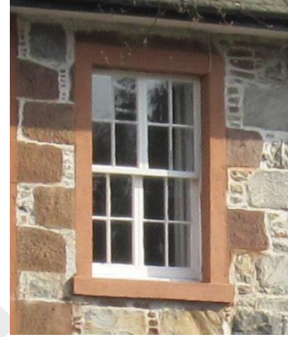
Fig. 44 8 over 8-pane sash and case window
