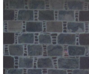
Fig. 41 Ladder pinning detail, lime mortar
