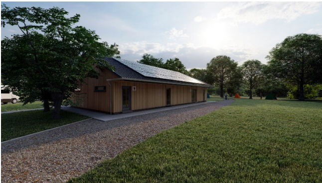
Fig 3. External view with solar panels
