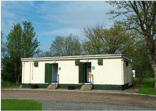
Fig 1. Existing toilet block
