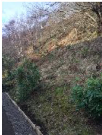
Embankment from below road
