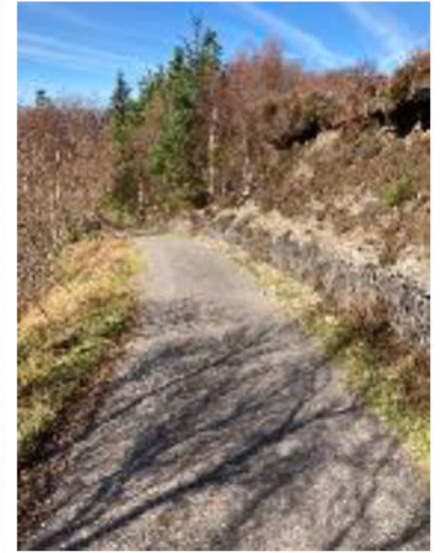
Narrow private access road leading down towards houses - erosion above
