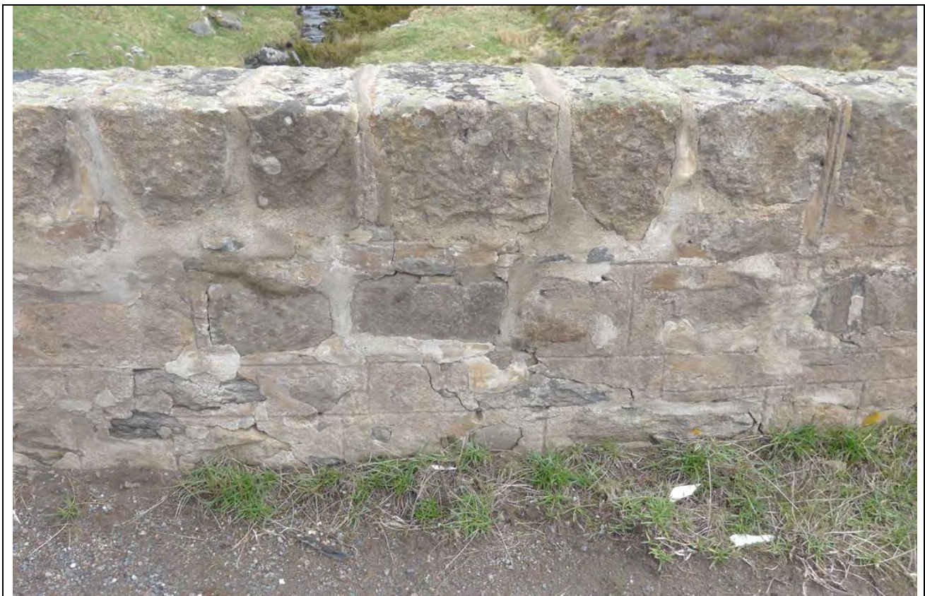
Photo 1 – Parapet elevation showing modern cementitious mortar over original lime mortar
