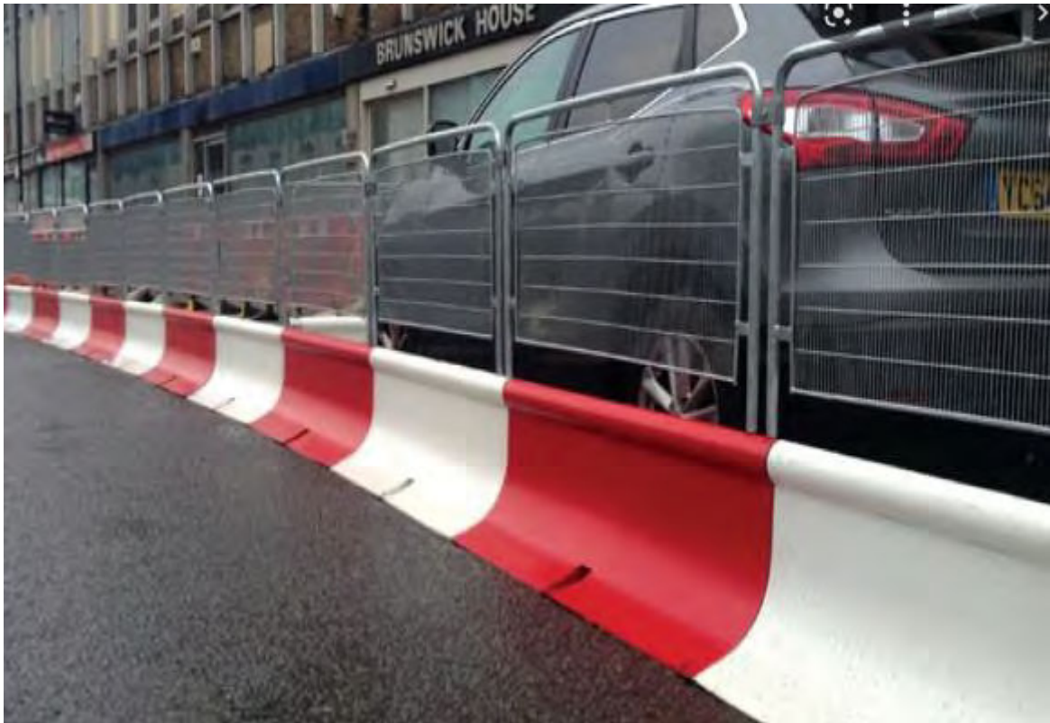
MASS barrier in place with pedestrian guardrail
