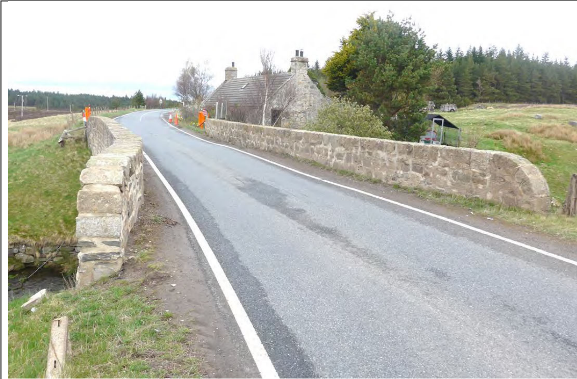
Photo 2 – General view of structure looking North
