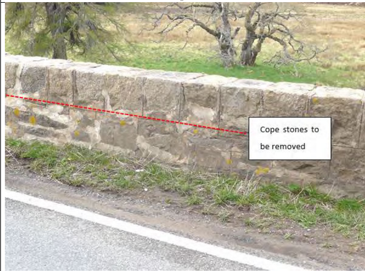
Photo 3 – Details of parapet with extent of wall to be taken down
