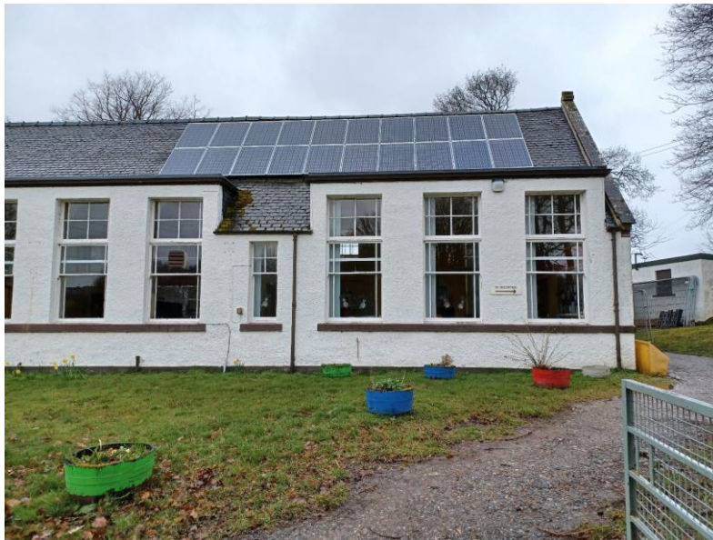
Figure 6: Existing 4kW solar PV system
