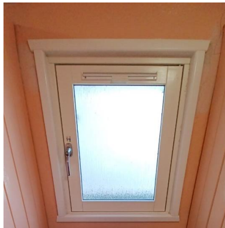
Figure 17: Tricklevents in double-glazed units
