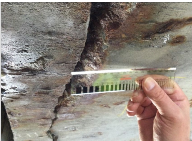
Photos: Ness Bridge (top), crack under the half-joint (bottom left), special investigation, 2023 (bottom right).
