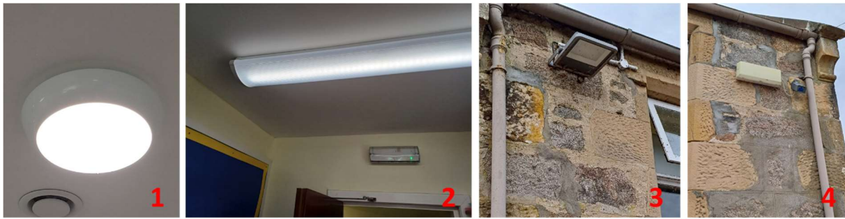
Figure 17: Typical Internal LED Lighting [1]; Typical Internal LED Strip Lighting [2]; External LED Lighting [3]; External Fluorescent Lighting [4]
