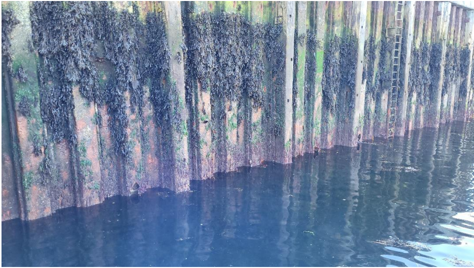
Photo 6: Sheet Piled Wall
