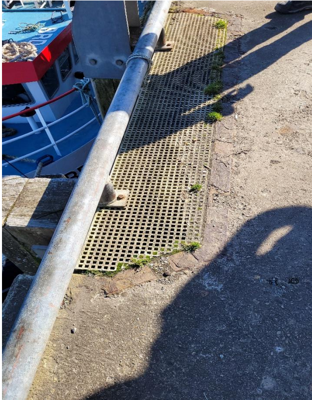
Photo 15: Fender Recess with Open Mesh Flooring
