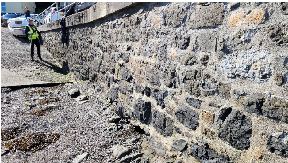
Photo 28: Repaired Sea Wall below Hotel at Beaumont Crescent
