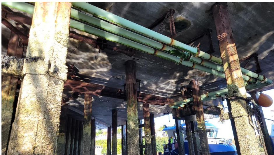
Photo 11: Redundant Pipework
