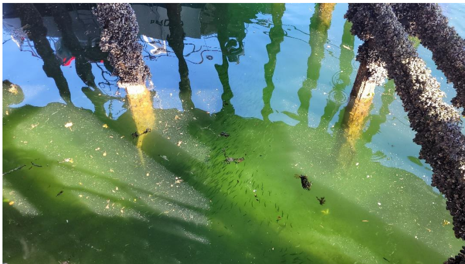
Photo 9: Rendhex Piles – Old Anodes
