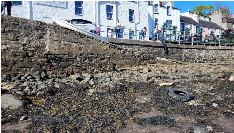
Photo 27: Beaumont Crescent Slipway
