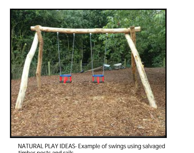
NATURAL PLAY IDEAS: Example of swings using salvaged timber posts and rails.
